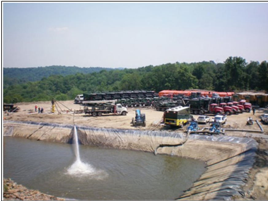
Figure 11. Temporary storage pond used in hydraulic fracturing
