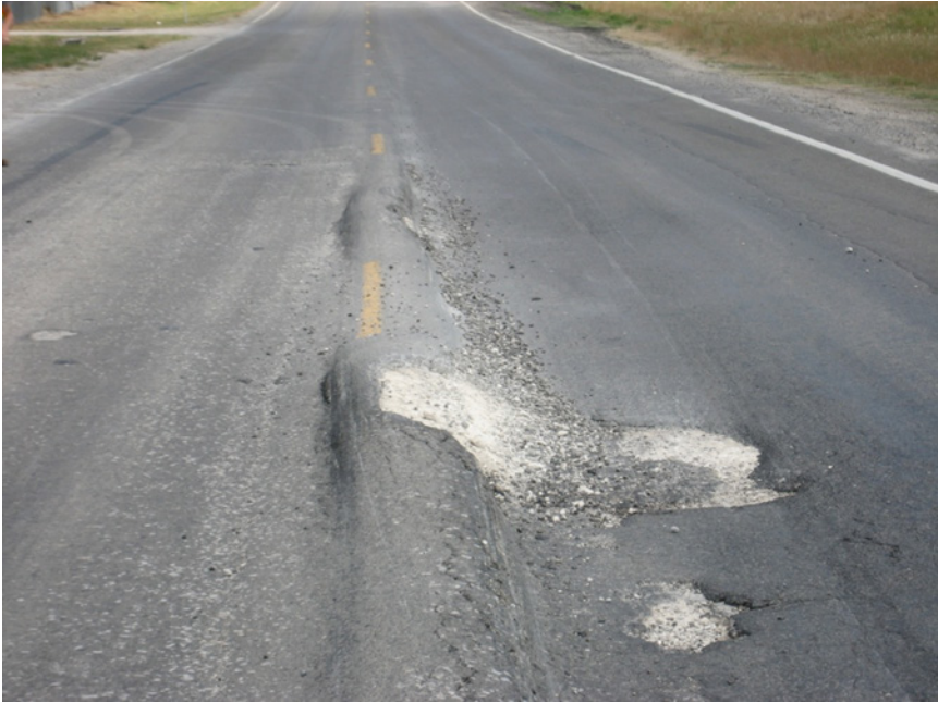
FIGURE 7-3 Pavement shoving, loss of surface (IH 35W – frontage road)
