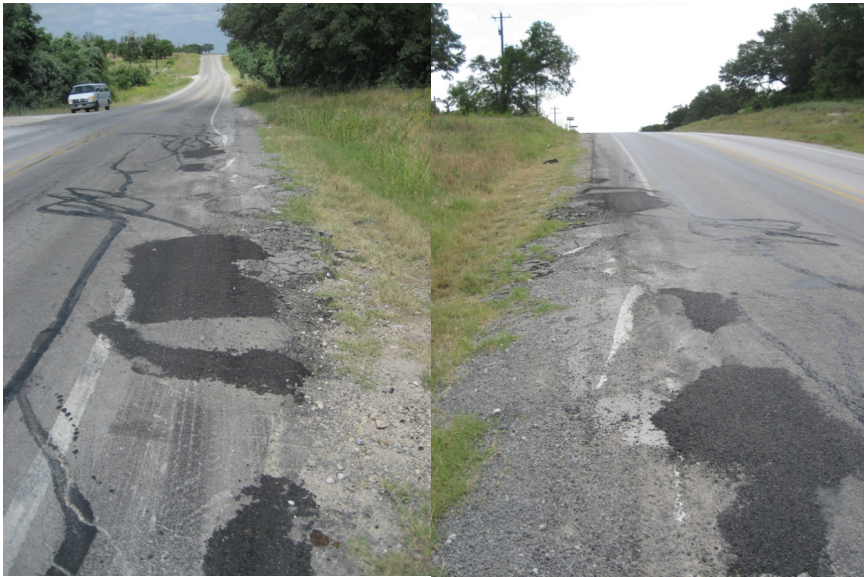
FIGURE 7-2 Shoulder patches on FM 2257 near saltwater disposal facility in Parker County.
